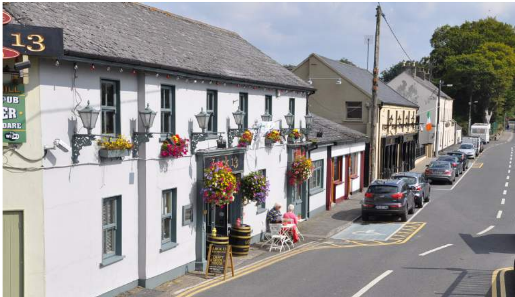
Top, separation of canal from buildings - dominance of vehicles in public realm bottom, pub/caf e attempting to expand into public realm
