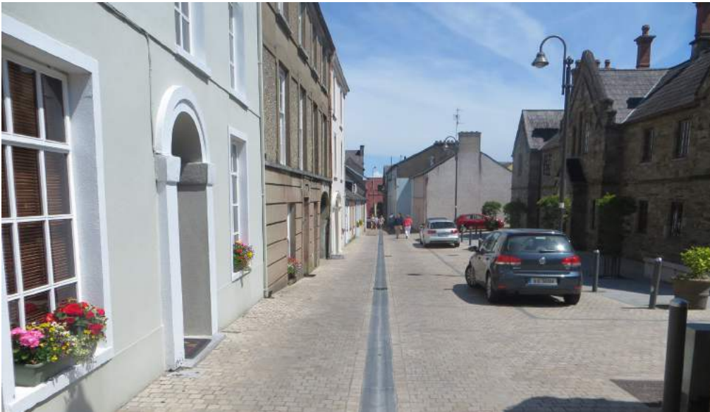
Shared surface in recent lane renovation in Youghal Co Cork. Sean McLoughlin/ Cork County Council
