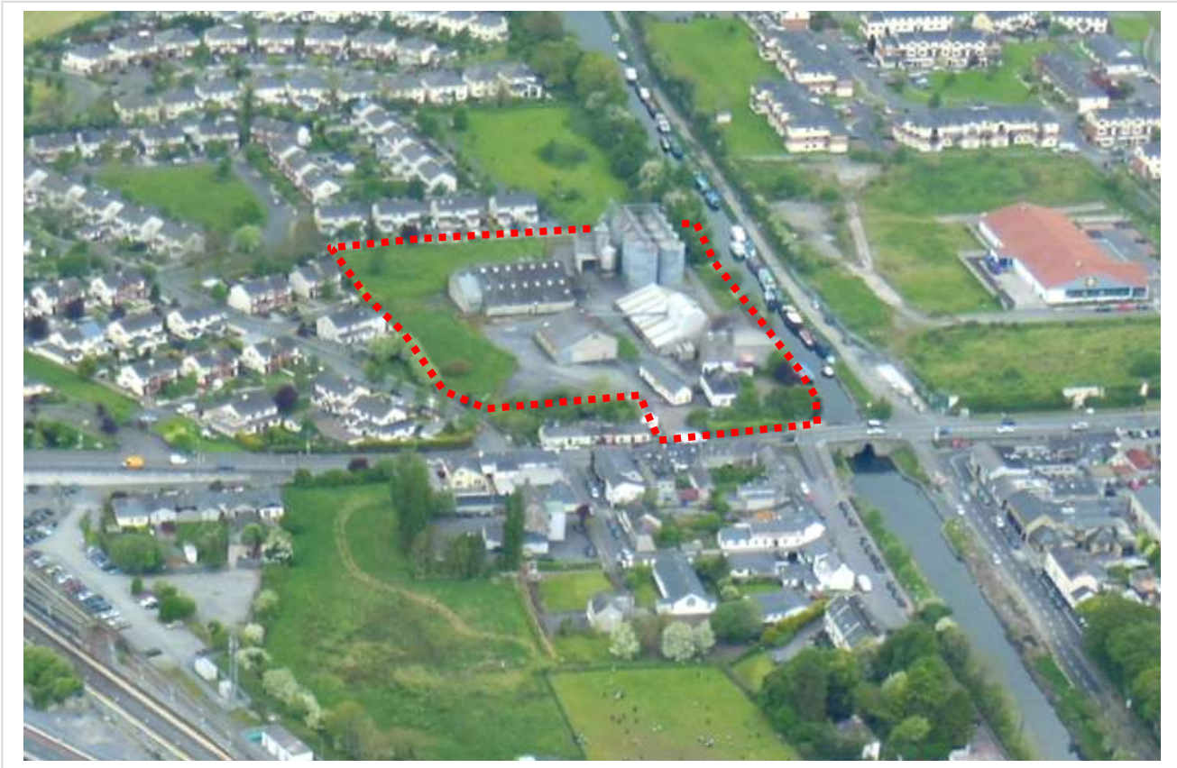
Aerial view of the site
