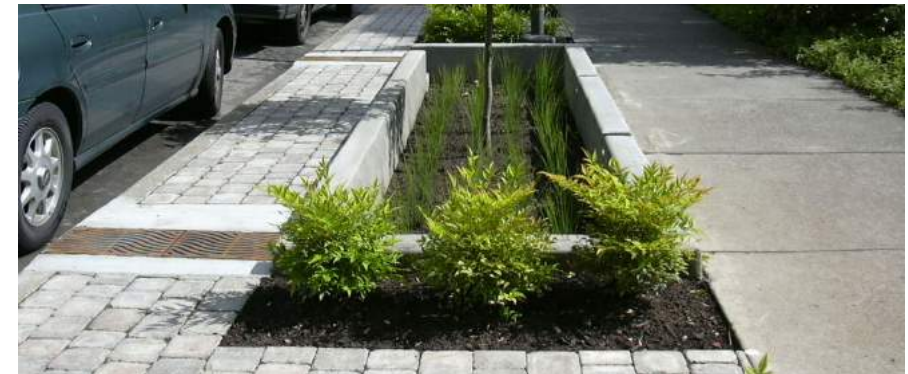
Top, high quality urban infill housing at the Triangle Swindon, UK by Haboakus. Below on street stormwater management of surface water, through vegetation
